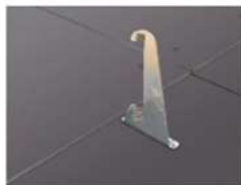
Snow guard support for grille-type snow guard
